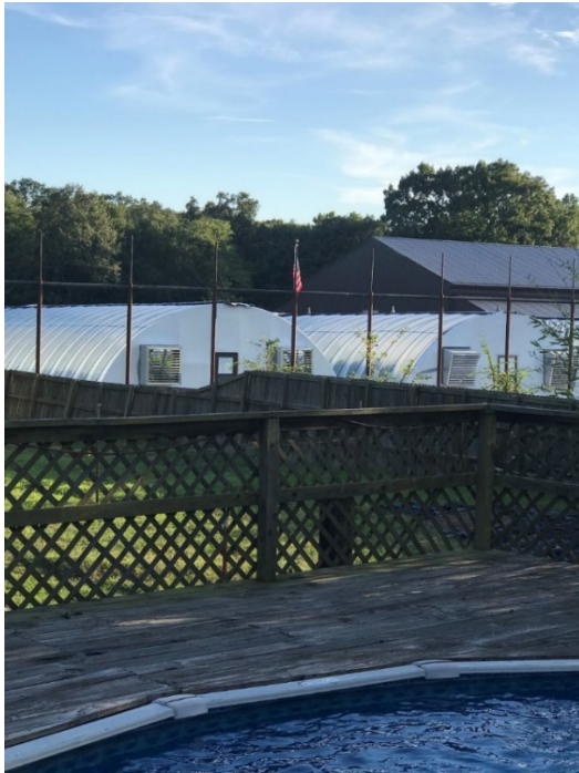
View of the unlawful marijuana operation from the Grants' pool deck.
