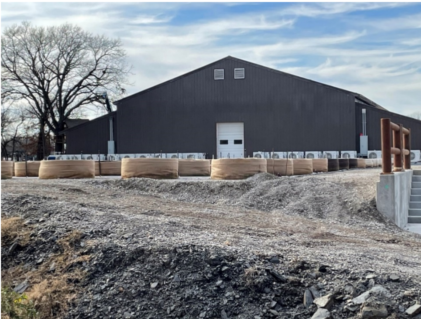
View of the marijuana grow outdoor pods situated on the backfill within the floodplain.
